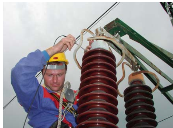
Figure 9. Ultrasonic testing on the hanging ceramic insulators of 440 kV transmission lines
